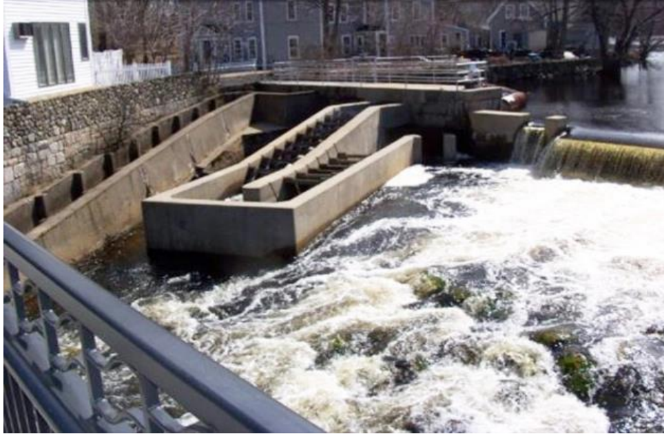
Caption: Neither the older abandoned fish ladder or the 1995 replacement have been very effective.
