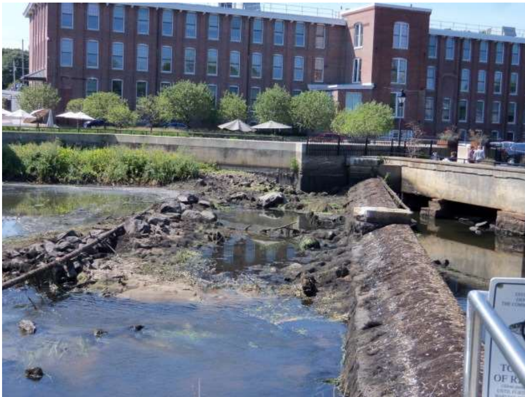
Photo 4: August 2016 Drawdown – The Ipswich River was drawn down behind the dam to better assess conditions in the impoundment, and an old gas line for the mill was exposed.
