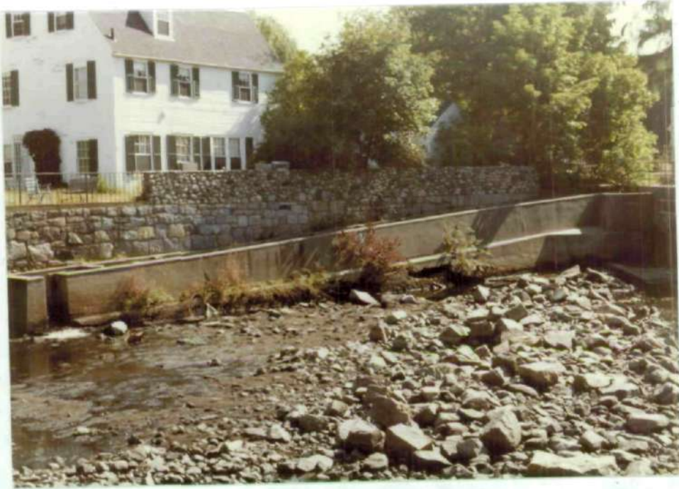
3. Fish ladder on right abutment of dam.
