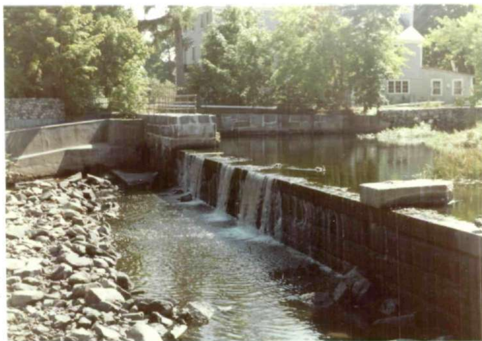
2. Downstream ashlar masonry face of dam.
