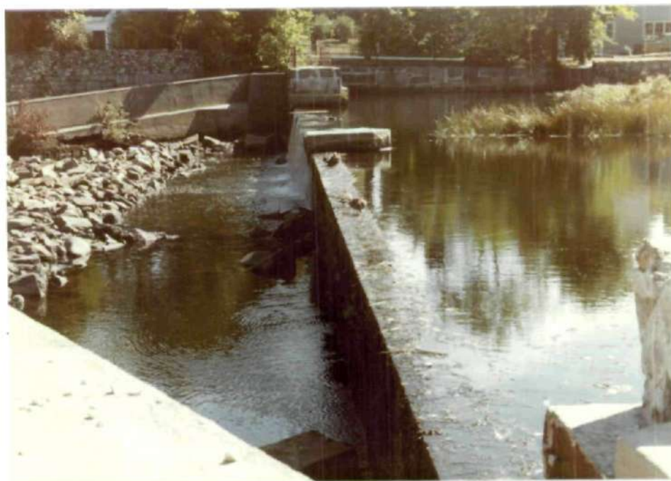
1. View along crest of dam from left abutment.
