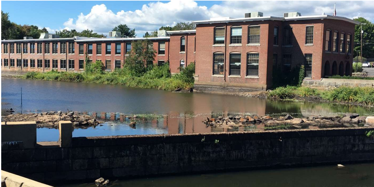
Photo 5: August/ September 2016 drawdown showing gas line removed.
