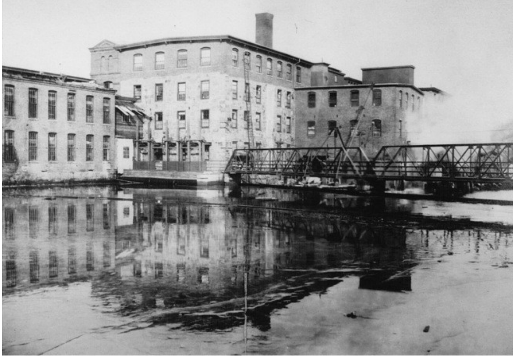
Photo 3: Ipswich Mills – View of the Mill just upstream of the dam and former pedestrian bridge circa early 20 th century. The shorter building in foreground is the current EBSCO facility. The larger building no longer exists.
