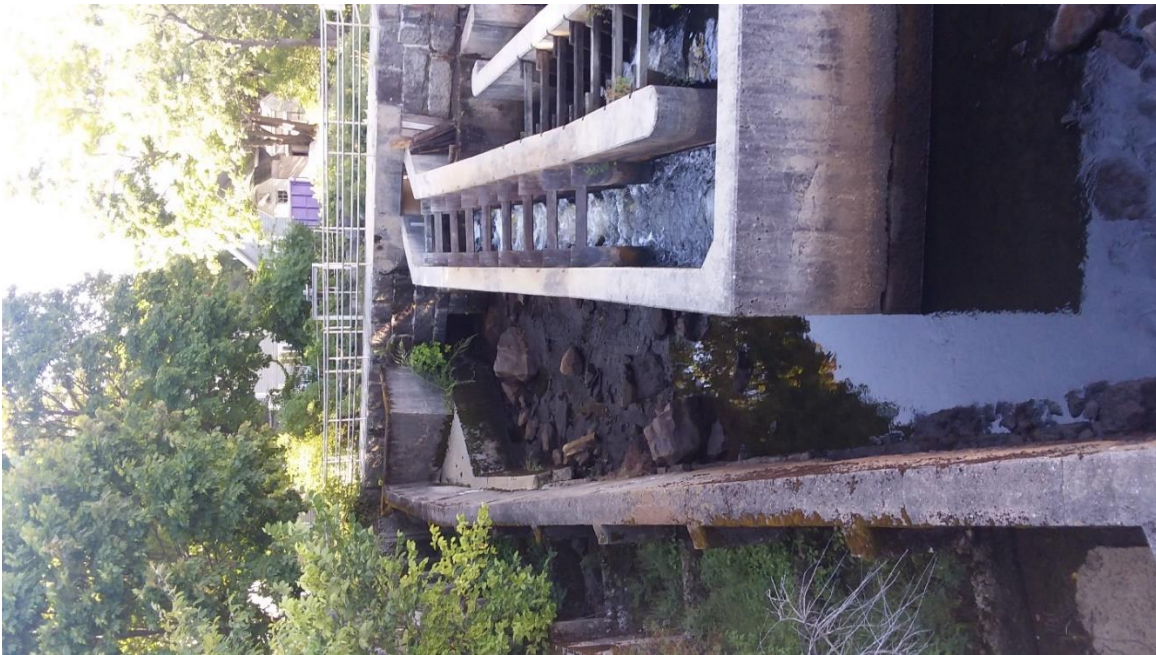
Photograph 8 – Low-level outlet discharge area between abandoned fishway and Denil fishway
