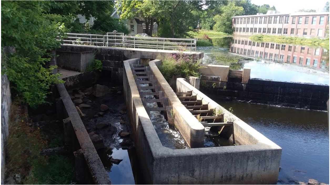
Photograph 1 – Dam, fishway, and right abutment looking from footbridge
