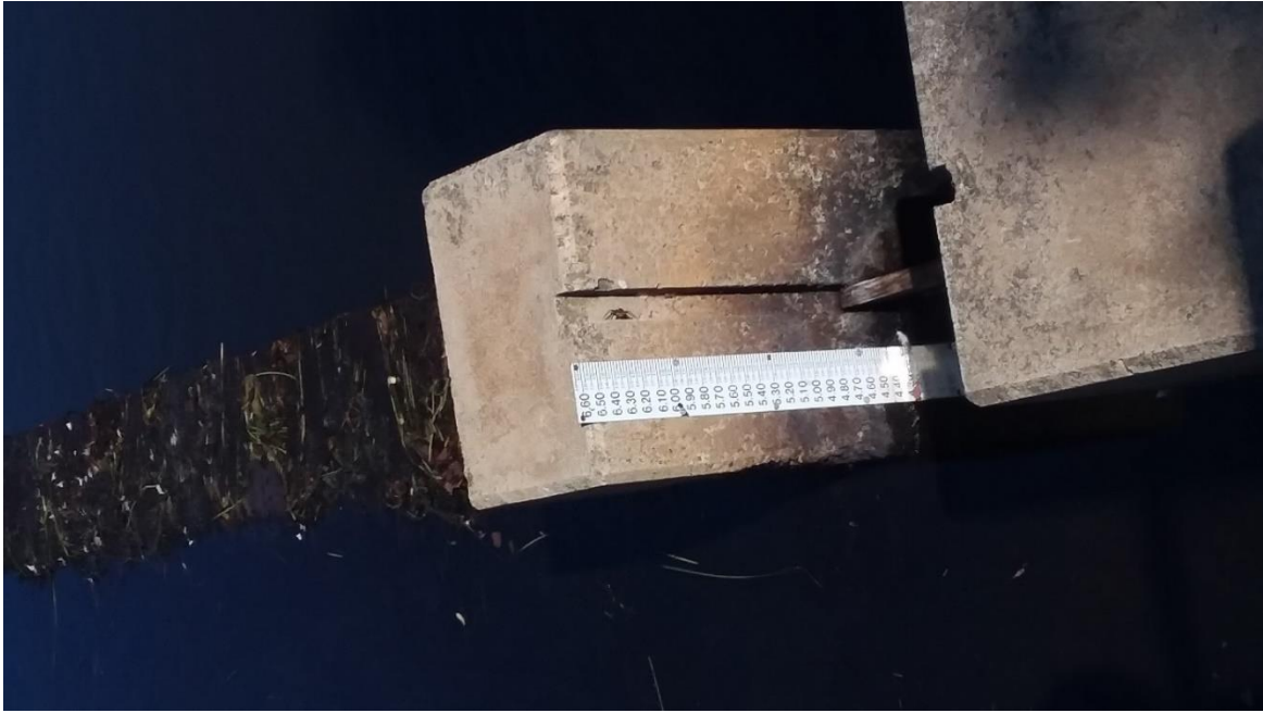
Photograph 19 – Staff gage at fishway attraction flow outlet looking from fishway viewing area
