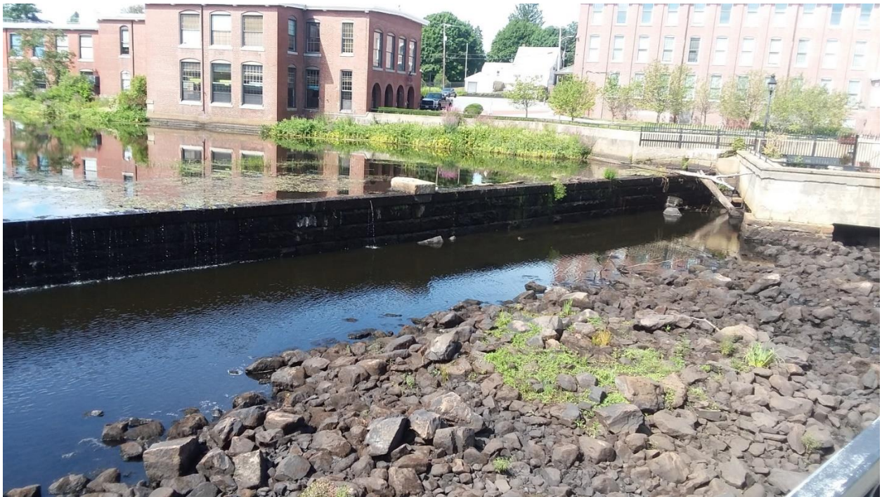
Photograph 2 – Dam and left abutment looking from footbridge
