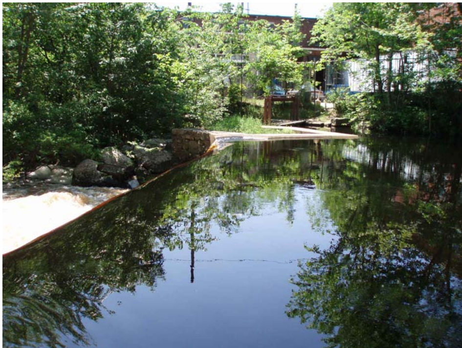
Photo 4: Spillway and Low-Level Outlet from Left Abutment
