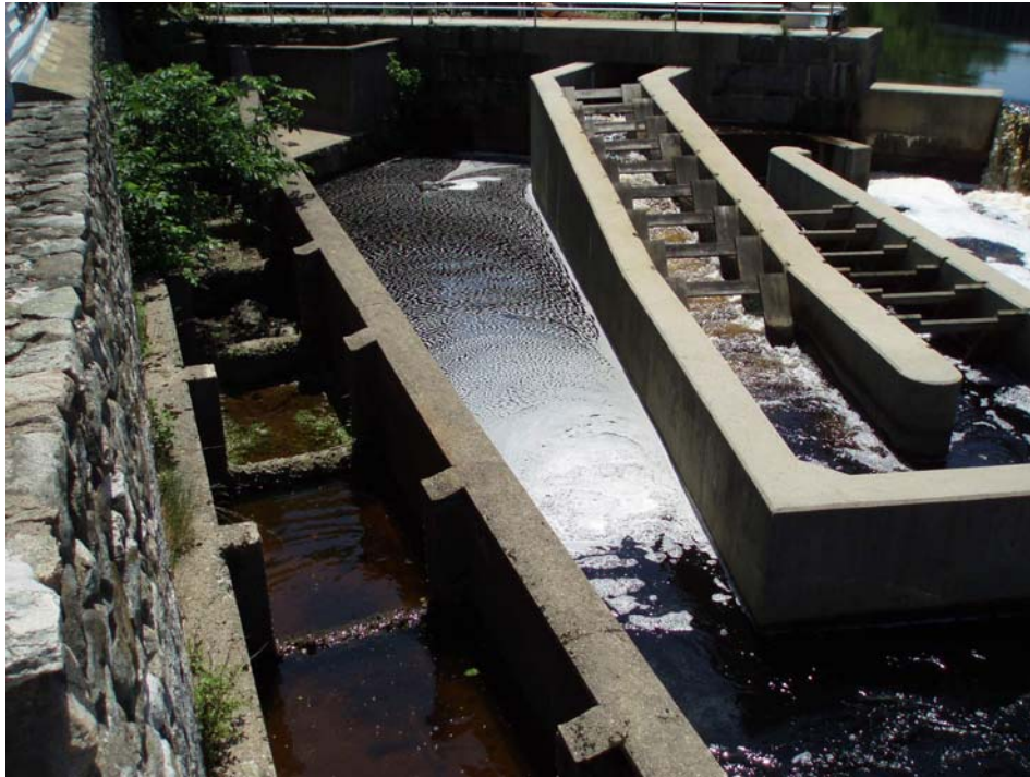
Figure 2: Abandoned Pools and Weir Fishpass (left) and Denil Fishpass (right)
