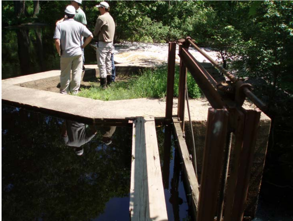
Photo 3: Low-Level Outlet and Spillway (background)
