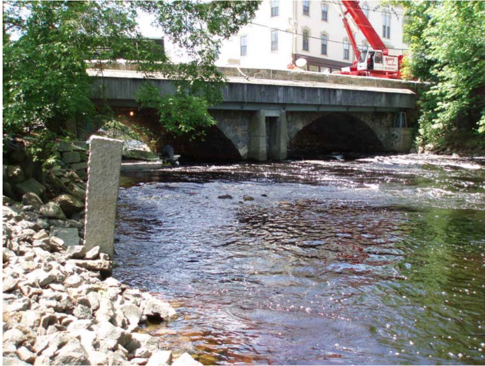
Figure 3: First Bridge over Ipswich River Downstream from EBSCO Dam
